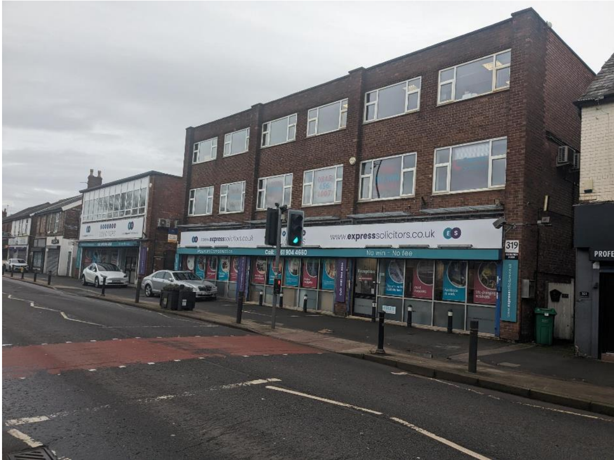
317-319 Palatine Road 'Resolution House' to the right 313-315 Palatine Road to the left
